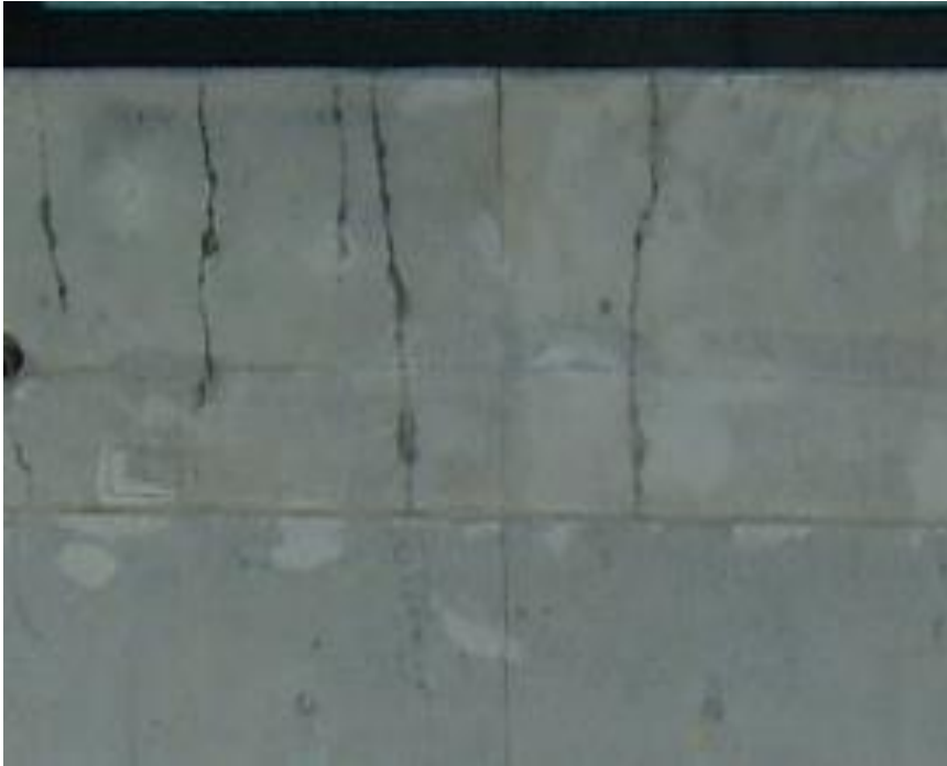
Thermal cracks in top of restrained wall
