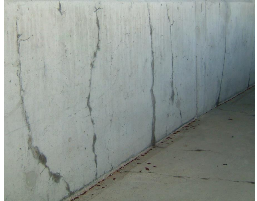
Thermal cracks in wall cast on existing structure
