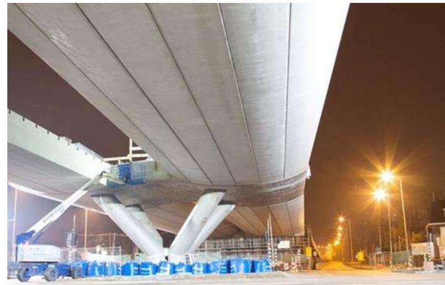
A lot is possible but to keep the economics in balance prefab has an influence on the esthetics of a structure – cross section shape and position of the supports.
