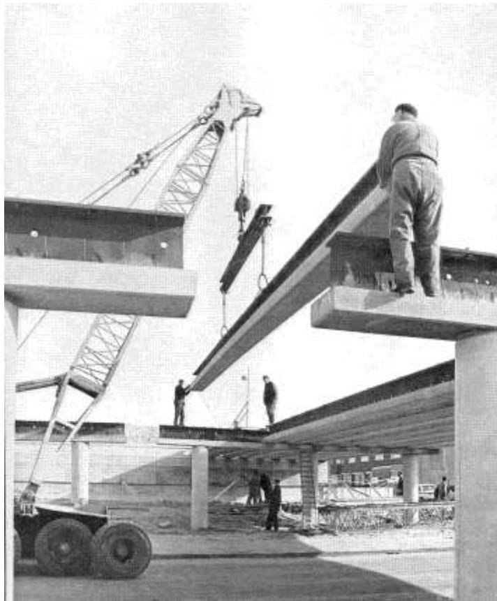
1970 span up till 37,5m with a height of 1260mm
